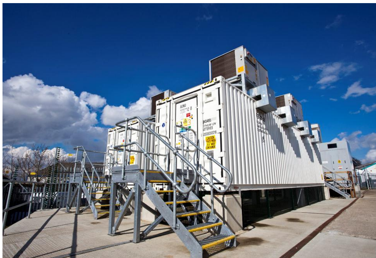
Image 1: 2.5MVA / 5MWh EES device at Rise Carr, Darlington, UK
