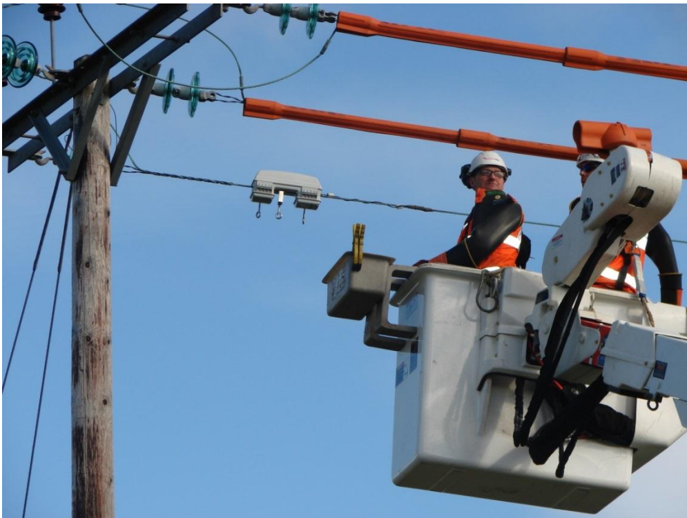
Figure 4 Installing On-Line Device using Hot Glove techniques
